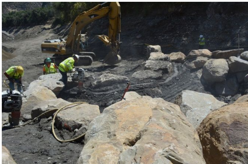
Construction of new step pools underway.
