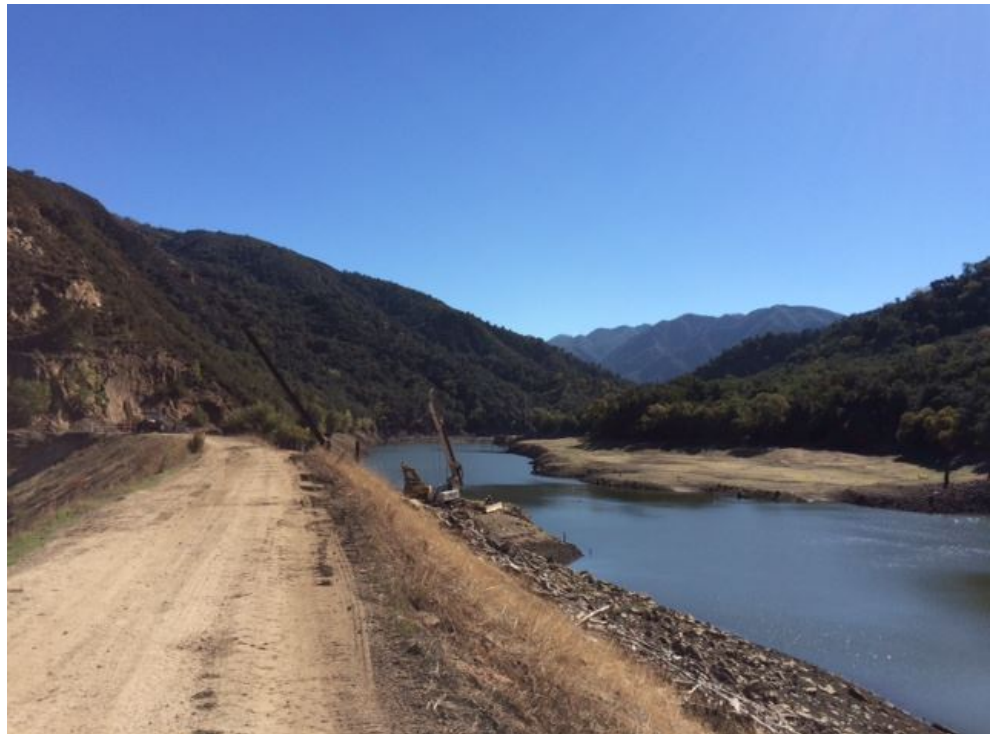
The Los Padres Reservoir where a smolt slide was recently installed to assist migrating steelhead in their downstream journey
